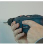
Using the appropriate drill bit, drill the marked holes
